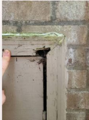
Wood decay noted at the wood pass through in the masonry chimney
