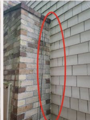
Wood decay next to the masonry chimney
